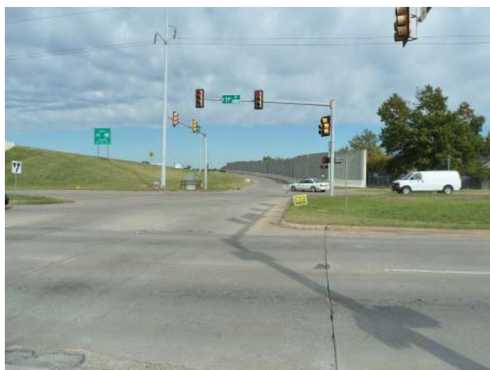
Lack of pedestrian crossings across East 21st Street
