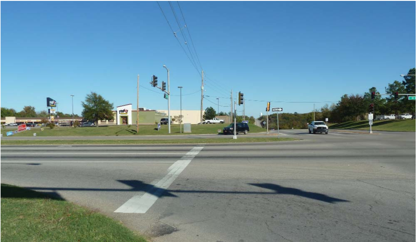
Existing photo looking east at the crossing of Highway 97 on 41st Street.
