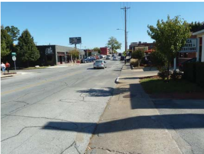
Lack of mid-block crossings along 15th Street
