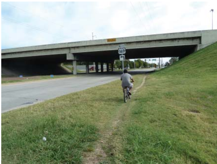
Lack of sidewalk under the Highway 169 overpass
