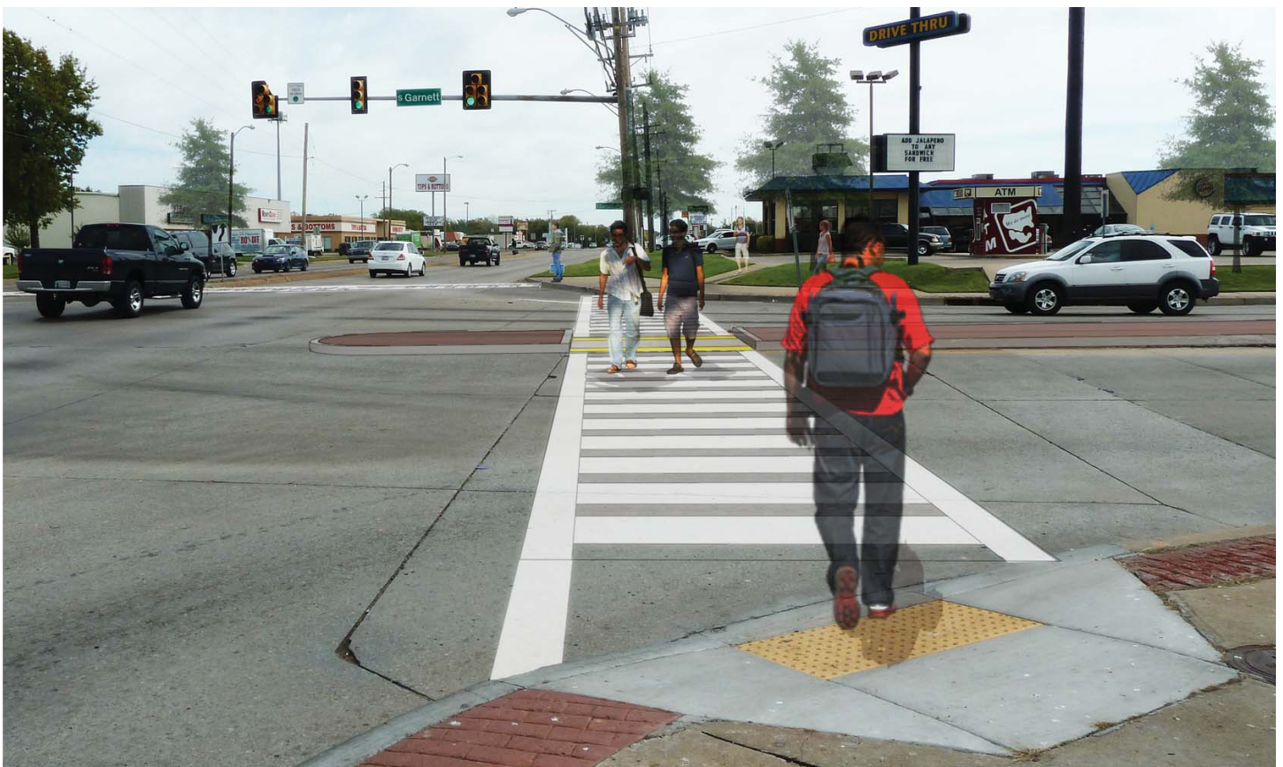
Conceptual photo-rendering of a high visibility crosswalk and raised refuge island median
