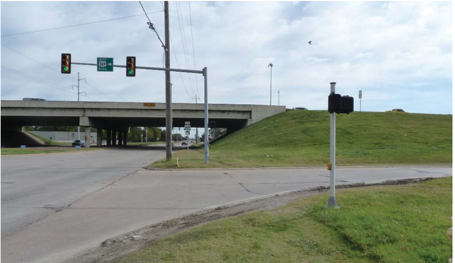
Existing photo looking east at the missing crosswalk at the crossing of the Highway 169 on ramp
