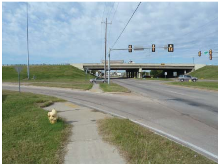
Lack of crossing at the Highway 169 off ramps
