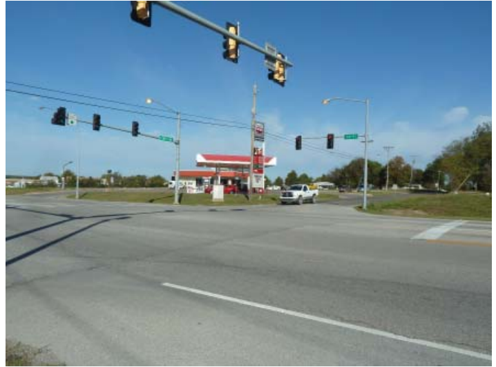
Lack of crosswalks and ramps at intersection.
