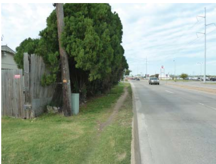
Lack of sidewalk along East 21st Street
