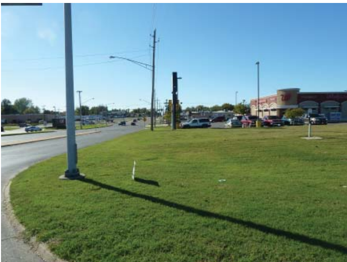
No sidewalks along E 41st St
